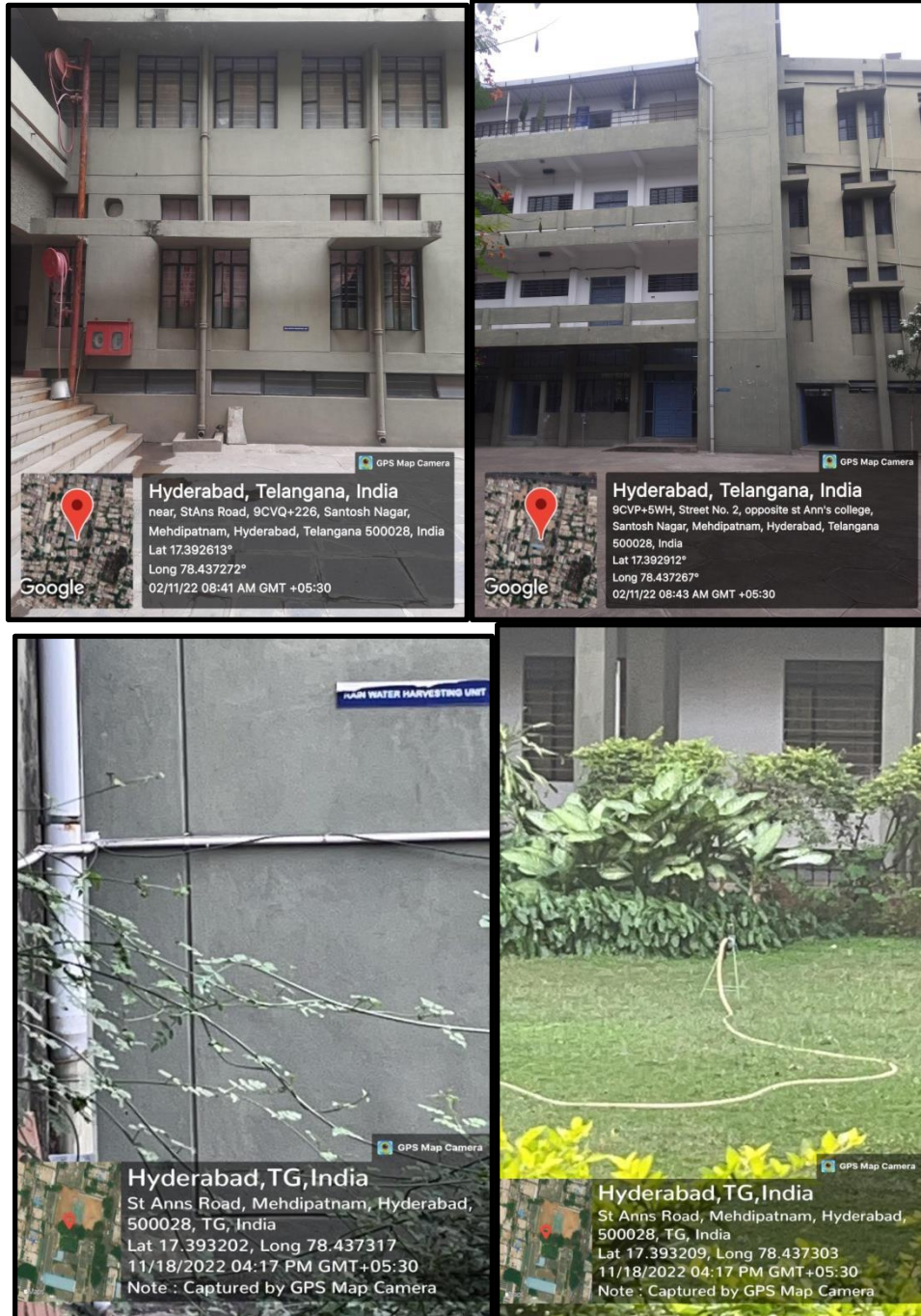
Rain water Harvest Pit
