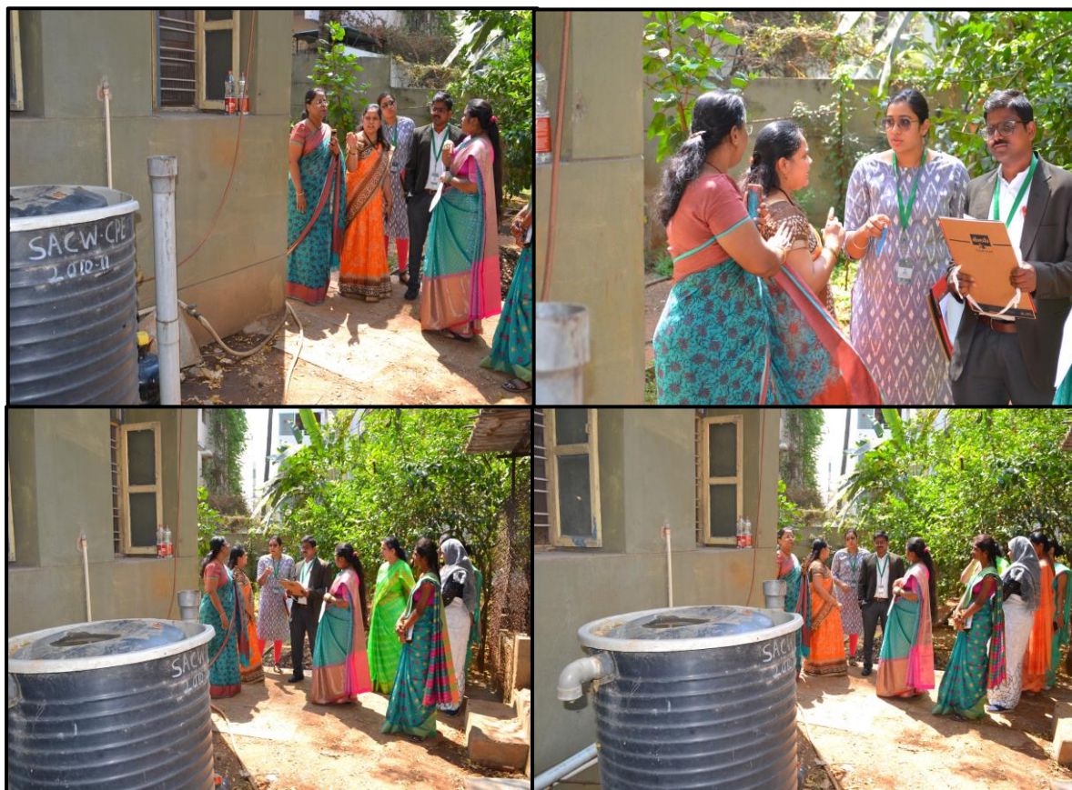
Biogas plant facility at the St. Ann's College for Women, Hyderabad, Telangana
