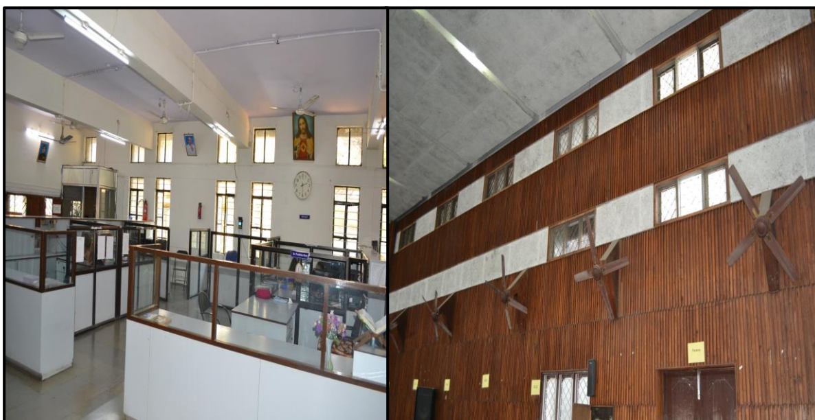
Sufficient Ventilation in St. Ann's College for Women Campus Buildings
